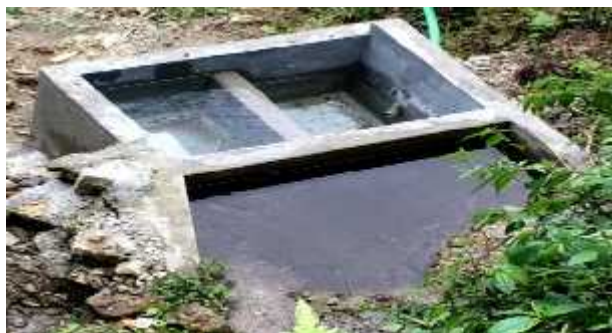
A newly Constructed Catchment and Distribution Tank
